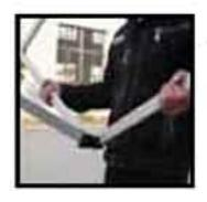
Next, grasp the lower "V" of the truss that you are facing. Lift up the shelter slightly and step back until the unit is halfway open.
